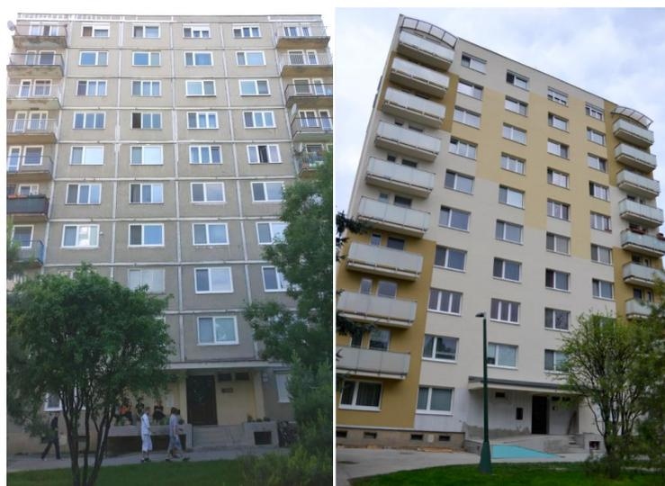
Figure 1. Residential building before and after renovation
